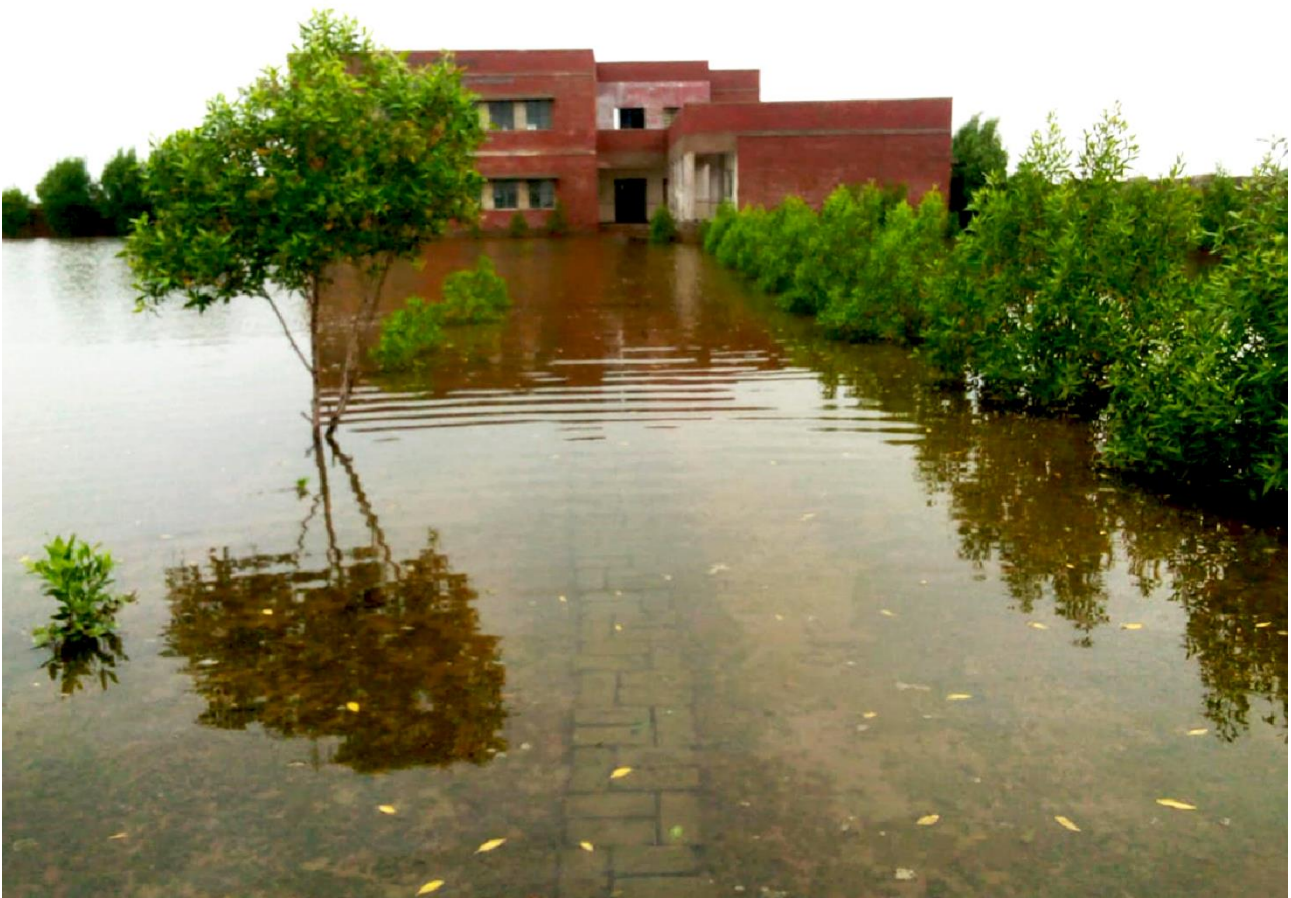
5.3. A school in Mirpur Khas submerged in water during the floods.
