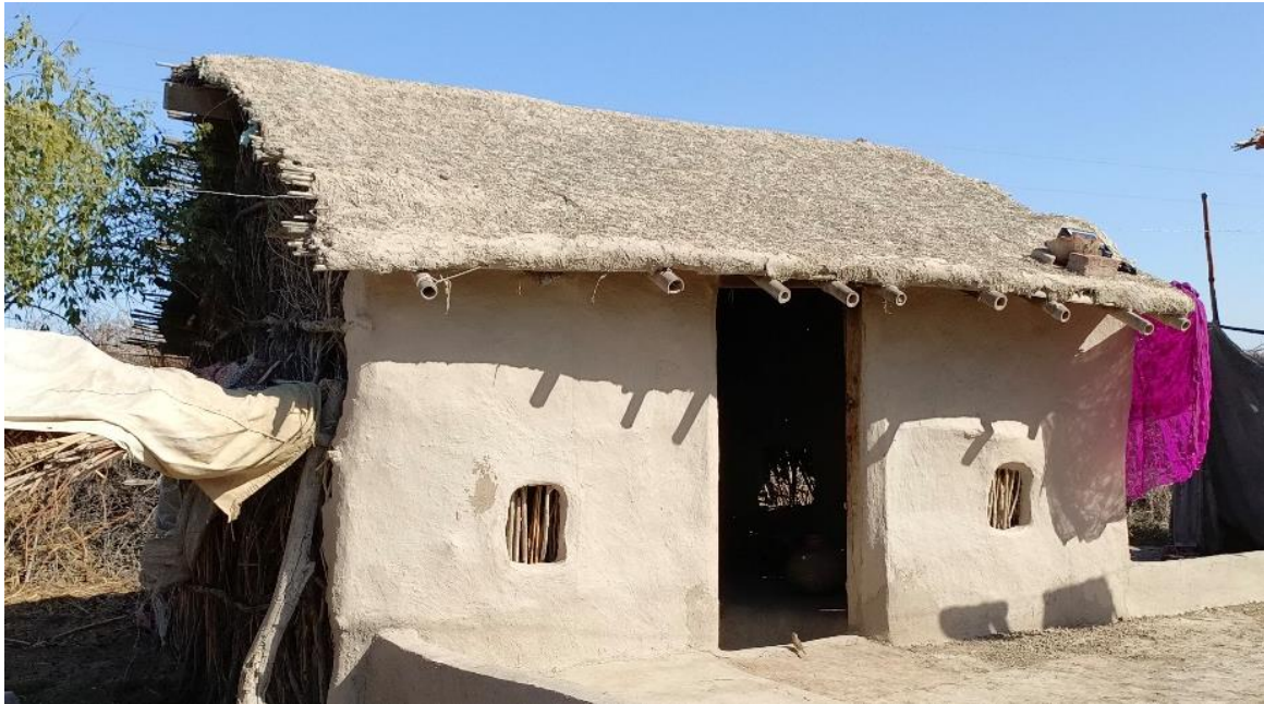
6.4. Kazi Academy, Mirpur Khas: one-room structure constructed by Reckitt, and covered in protective mud-plaster by the locals.
