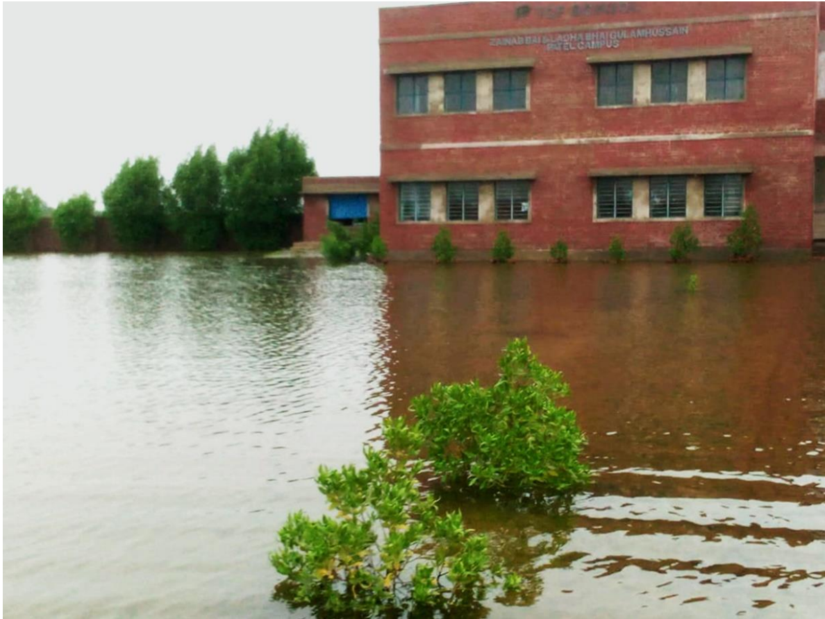
8.1. TCF school and surrounding roads submerged in water
